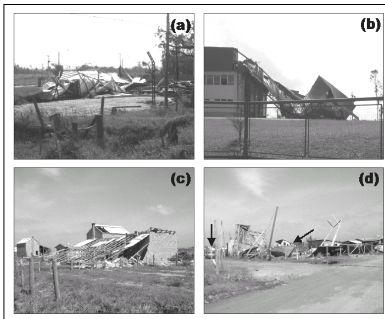
Figure 5 – Types of damages caused by wind force on sheds: (a and b) total and partial collapse of metallic sheds; (c) partial collapse of tobacco warehouses; and (d) total collapse of a shipyard.
