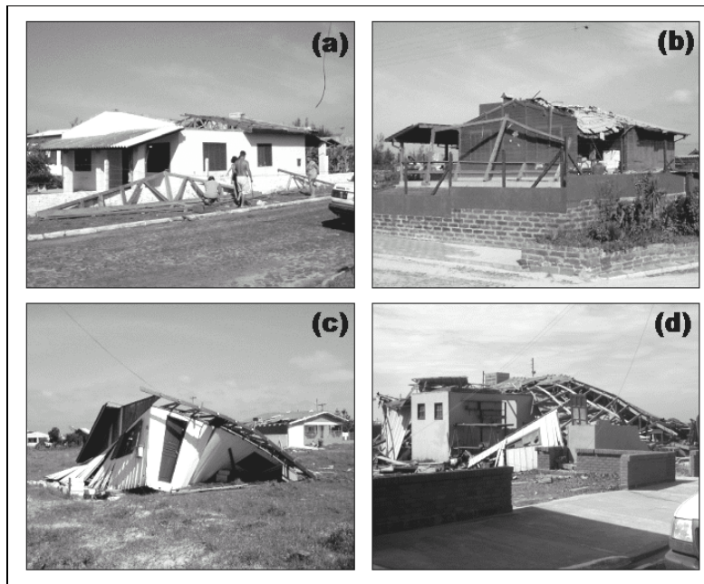
Figure 4 – Types of damages caused by wind on residences: (a) total roof failure; (b) partial roof failure of a non-engineering wood house; (c) total destruction of a non-engineering wood house; and (d) total collapse of a masonry house.
